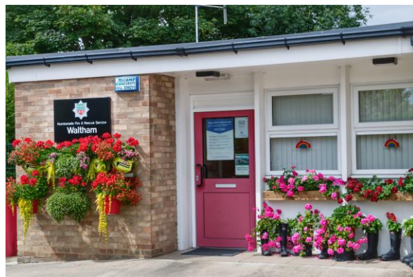
The Fire Station at Waltham
